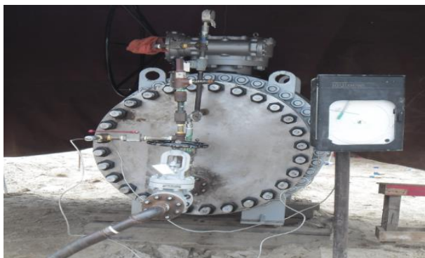
Fig.23: Hydrostatic test arrangement
